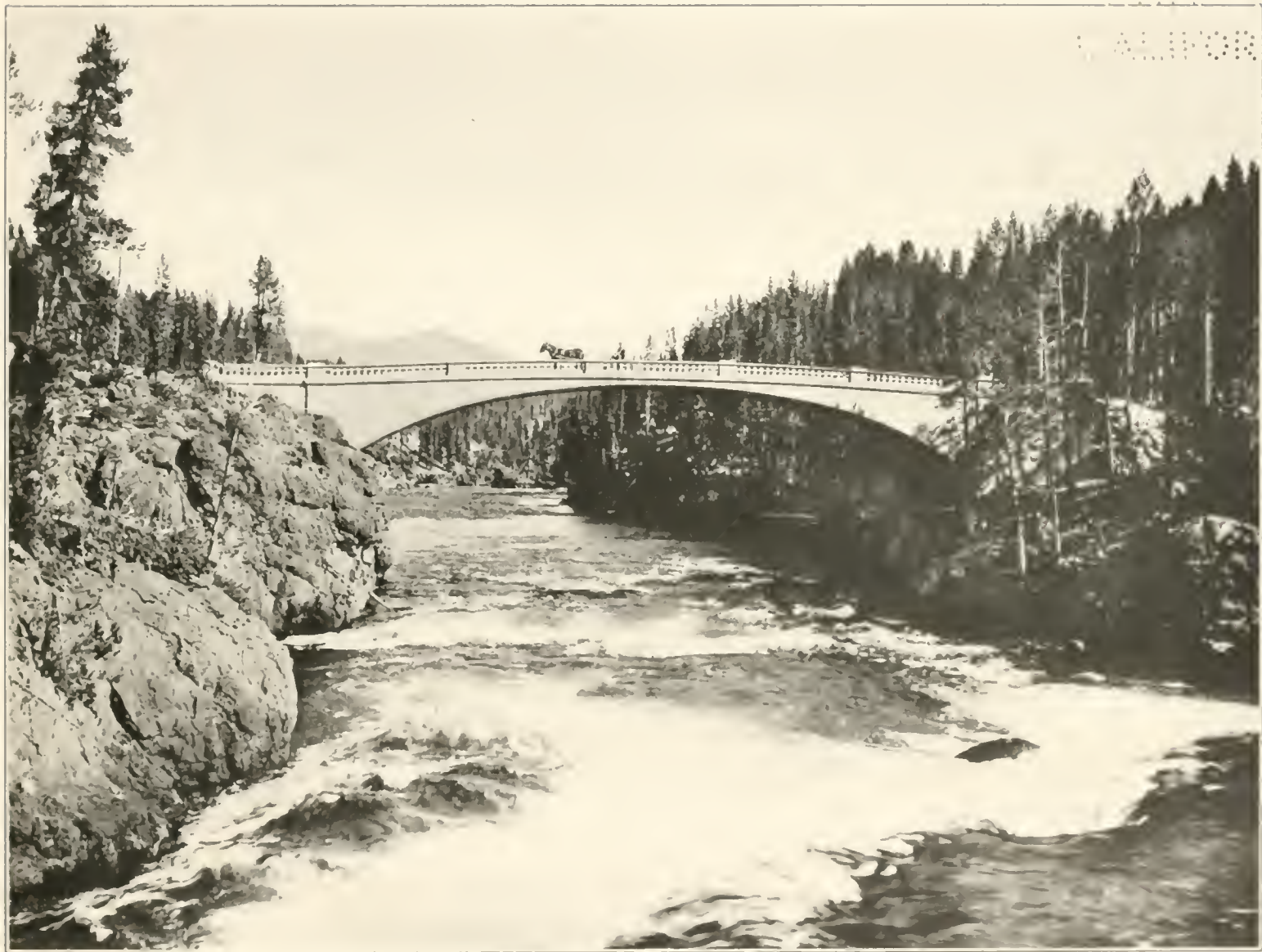
YELLOWSTONE BRIDGE — ABOVE THE UPPER FALLS
